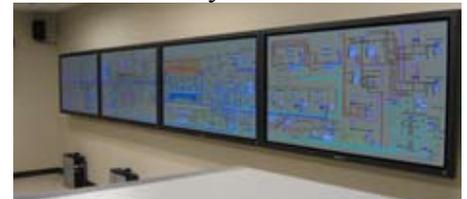
*Kongsberg's Big View® has replaced the company's older mimic panels, and offers reconfiguration flexibility for different engine models, as well as other visualization applications. The GLIMTC configuration uses four 65" Panasonic plasmas. Photo courtesy of Håkon Dyrvik*
