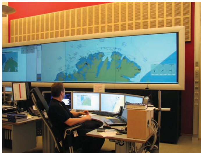
▲ The operator has four screens. The two to the right are the VTS screen and actual traffic. The two screens to the left are the OSS and an administration PC
