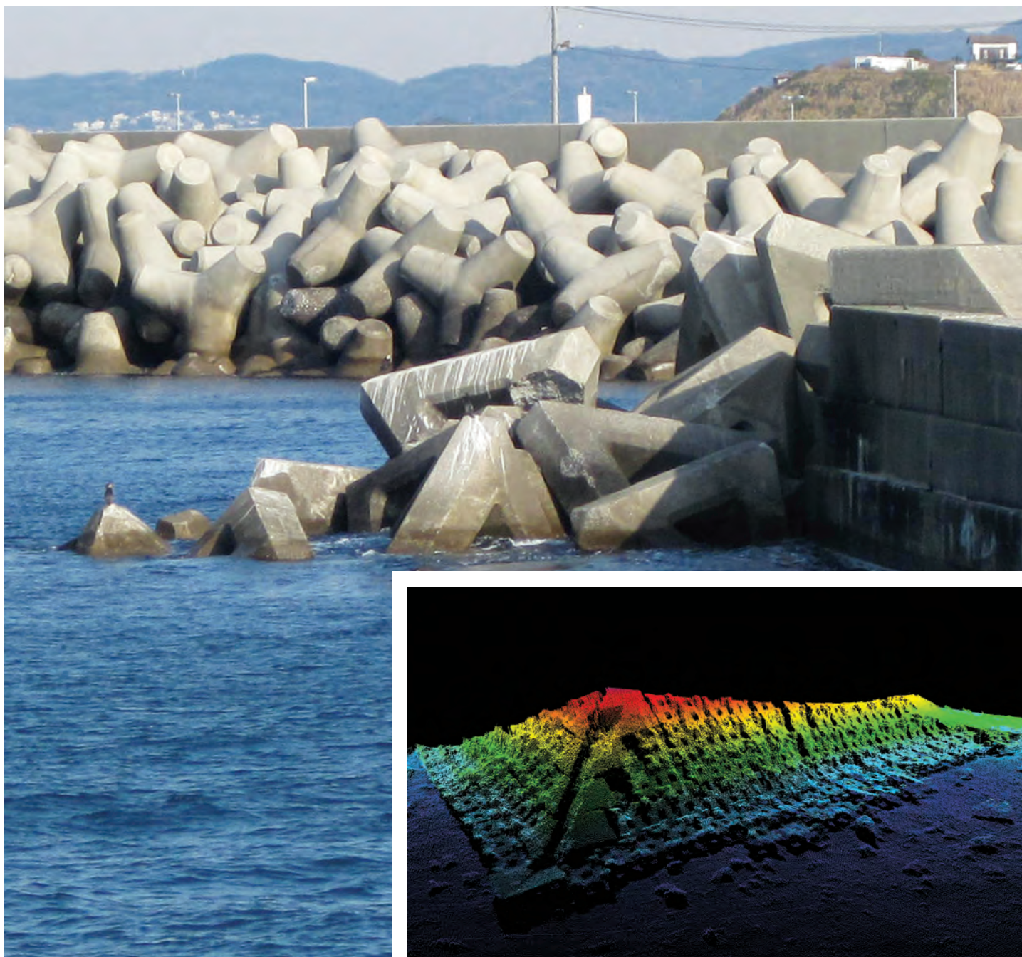
Getting the full picture Seapath with MRU 5+ as the INS component, achieves state-of-the-art results when used in conjunction with the KONGSBERG EM2040 multi-beam echo sounder for surveying submerged pier elements.
