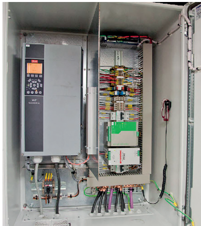
Control cabinet with frequency converter
