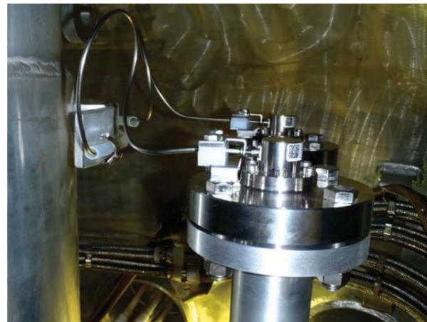
Figure 11: Dual radar antenna inside tank (example)
