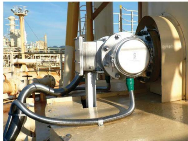
Figure 10: Side penetration with dual radar configuration (example)
