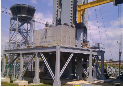
HRAS delivery platform and RAS mast at HMS Raleigh
