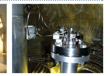
Figure 10: Side penetration with dual radar configuration (example)
